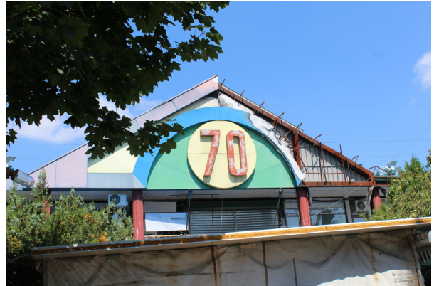
Markthalle in Block 70
